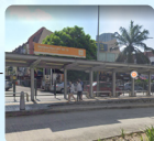
SS15 LRT STATION (GATE B BUS STOP)
