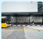
TAYLOR'S LAKESIDE CAMPUS (BLOCK B)
